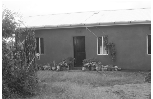
Refurbished Teacher's House at Geytighi Primary School
